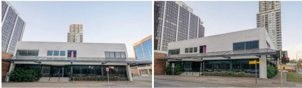
23-27 Macquarie Street, Parramatta
